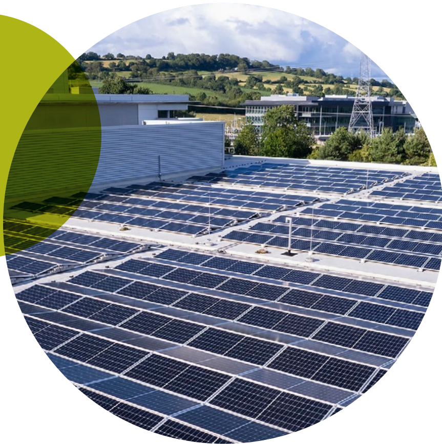
Solar panel installation Gilead Cork, Ireland
